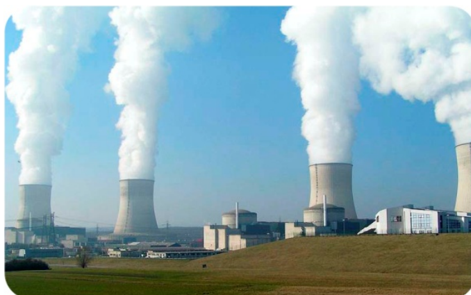
Figure 6 - A nuclear power plant - the smoke seen is steam from cooling towers.
